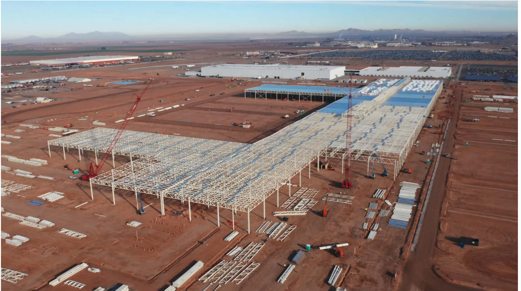
Note (1): Photograph of expansion project as 02/25/2022.
